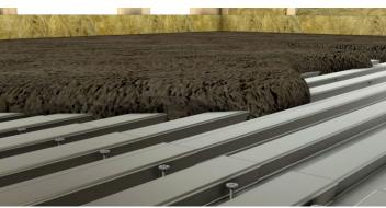
The screws / nails are placed in each corrugated bottom along all beams. The top of the screw / nail should align with the top of the sheets. Cast as described on page 4.
