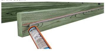
Apply the sealant below the line on the beams.
