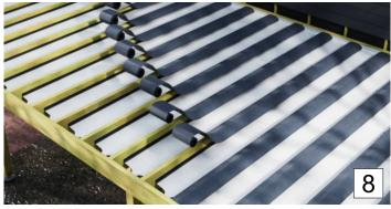
Roll out TIL-TAK asphalt felt on top of all the joists.
