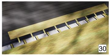
recommend removing 2 deck boards for dry transition and inspection/cleaning of debris.
