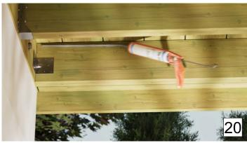
Apply the TIL-TAK caulk below the line along the joist.
