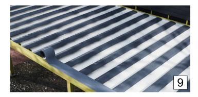
Also use TIL-TAK asphalt felt on top of the rim joist to leave it dry underneath. Shape
