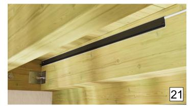
Press the PVC tracks along the line. The TIL-TAK caulk must appear on all sides of the pvc tracks.
