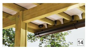
The tongue will function as downspouts, leading water into the gutter.
