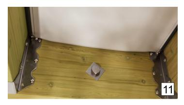
Stretching the canvas is needed. Attach a screw through the track under the canvas on each side, close to the wall ledger. Stretch the canvas on each side on the outer end
