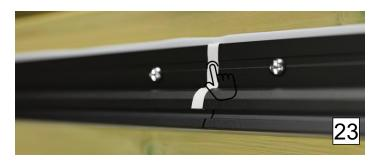
Apply caulk above the groove of each track joint. Then smoothen the caulk with your
