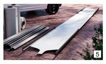
Slide the PVC tracks on to each side of the canvas while it is still on ground level. Make sure that the print on the canvas is facing up. Make a mark at the very top of the joist
