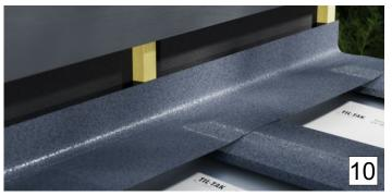
the asphalt felt as illustrated against the wall on top of the wall ledger, to maintain a dry transition.
