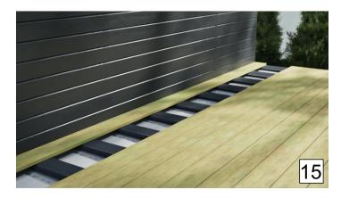
Start installing the deck boards from the wall, working your way outwards. Leave a
