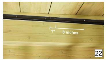
Fasten with TIL-TAK Light screws every 8 inches. Max 1 inch from each end of the track.
