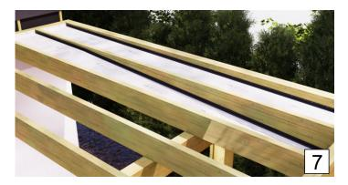
Install the PVC-tracks with the canvas to the joists along the chalk line. Fold the trimmed end up, and staple to the ledger board.
