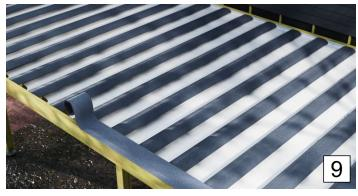
Also use TIL-TAK asphalt felt on top of the rim joist to leave it dry underneath.
