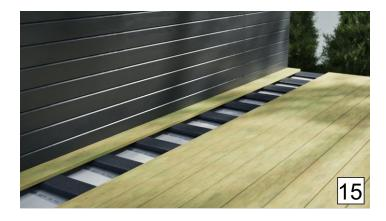
Start installing the deck boards from the wall, working your way outwards. Leave a space of 2 deck boards...
