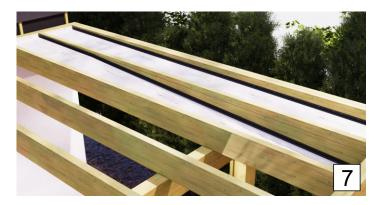
Install the PVC-tracks with the canvas to the joists along the chalk line. Fold the trimmed end up, and staple to the ledger board.
