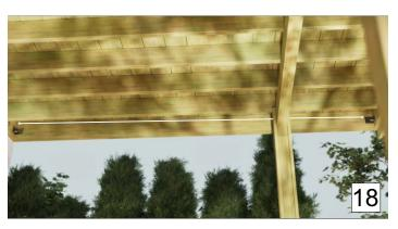
As with new construction, draw a straight line from inside to outside, with a minimum drop of  $\frac{1}{2}$  inch per 4 feet (ref. pict. no.6)
