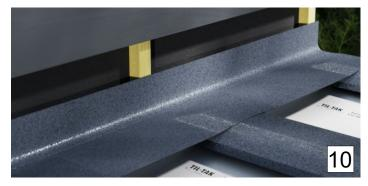
Shape the asphalt felt as illustrated against the wall on top of the wall ledger, to maintain a dry transition.
