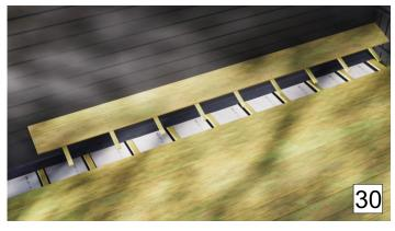
Ref. pict. no 10 and 16, we recommend removing 2 deck boards for dry transition and inspection/cleaning of debris.
