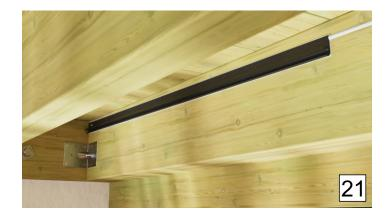
Press the PVC tracks along the line. The TIL-TAK caulk must appear on all sides of the pvc tracks.
