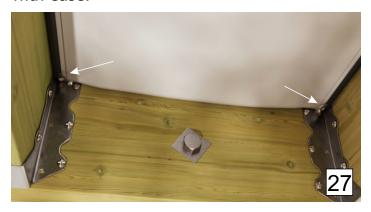
Stretching the canvas is needed. Attach a screw through the track and canvas/rope on each side close to the wall ledger.
