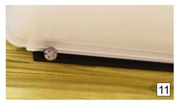
Stretching the canvas is needed. Attach a screw through the track under the canvas on each side, close to the wall ledger.
