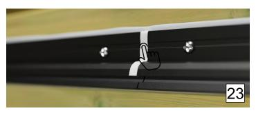
Apply caulk above the groove of each track joint. Then smoothen the caulk with your finger.
