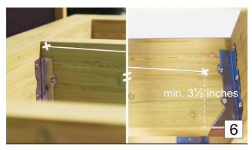
Make a mark at the very top of the joist towards the wall. Make an additional mark at the other end of the joists, min. 3½ inches from the bottom. Snap a chalk line between the 2 points. Minimum drop: ½ inch per 4 feet
