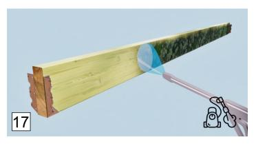
Clean the joists properly using a pressure washer, for the sealant to adhere. All dirt must be removed before the TIL-TAK caulk is applied.
