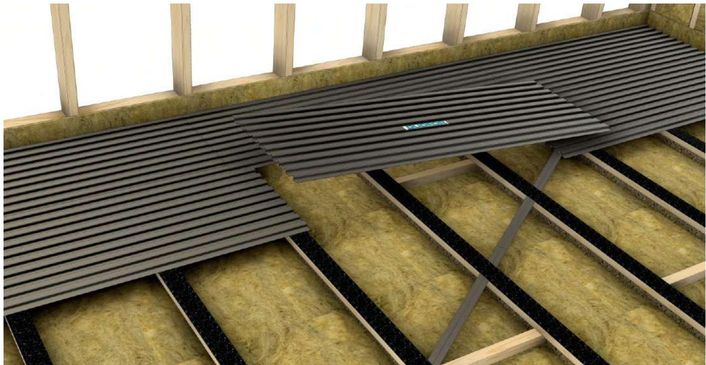
Cutting and adjustments can be made both with a jigsaw or a circular saw with hard-metal blade. If the waste is too short to be used, it is better to only shift the plates with a larger overlap.
